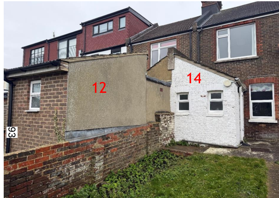
Fig 3.0 Photo of existing rear elevation and neighbouring property no. 12
