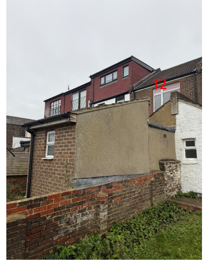
Fig 1.2 views towards neighbouring property no. 12
