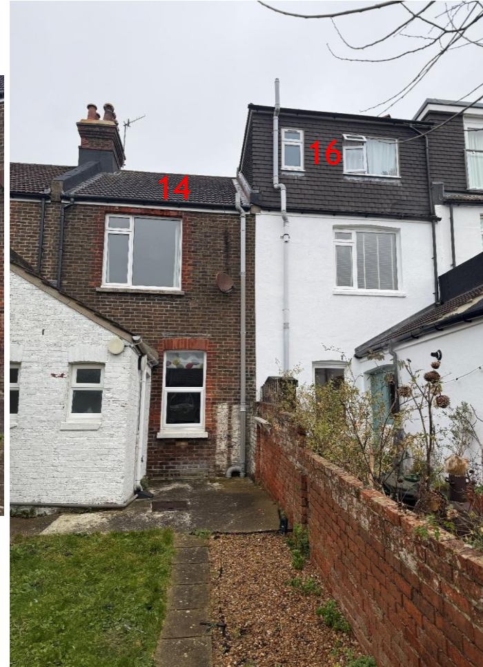
Fig 3.1 Photo of existing rear elevation and existing rear extension
