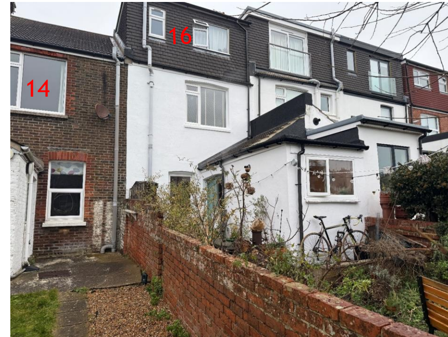
Fig 3.2 Photo of existing rear elevation and neighbouring property no. 16
