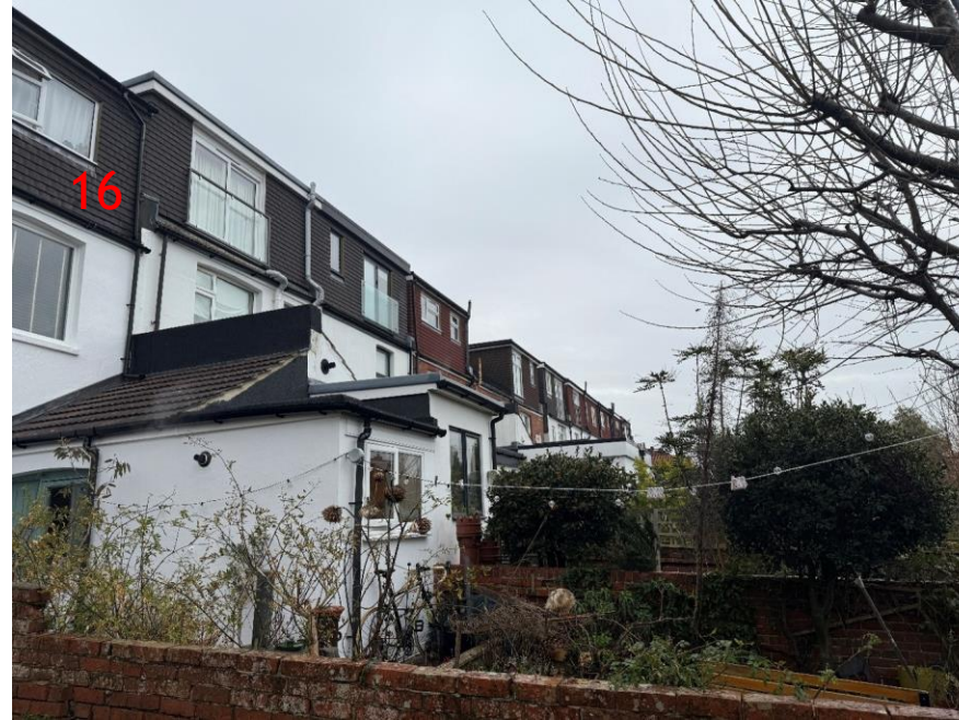
Fig 1.1 views towards neighbouring property no. 16
